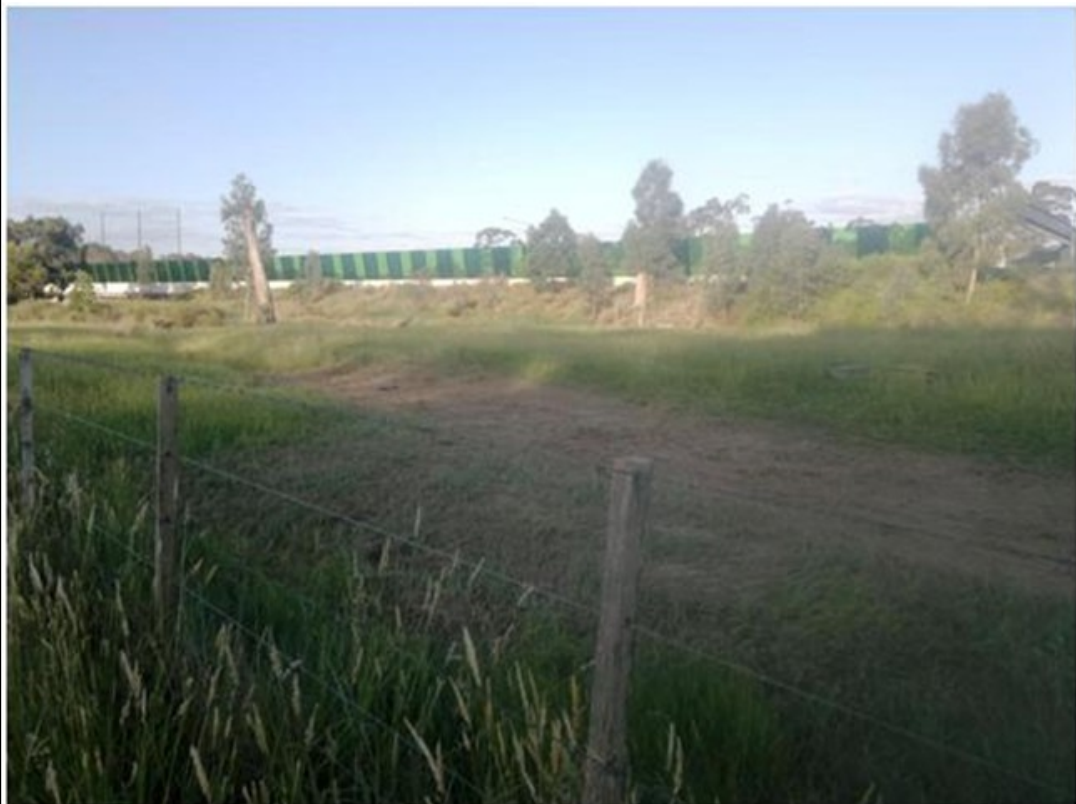
Filled in spoon drain now allowing the natural flow of water back into Winton Wetlands.
