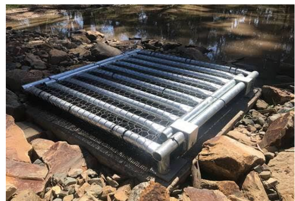
Temporary pitfall drain cover
